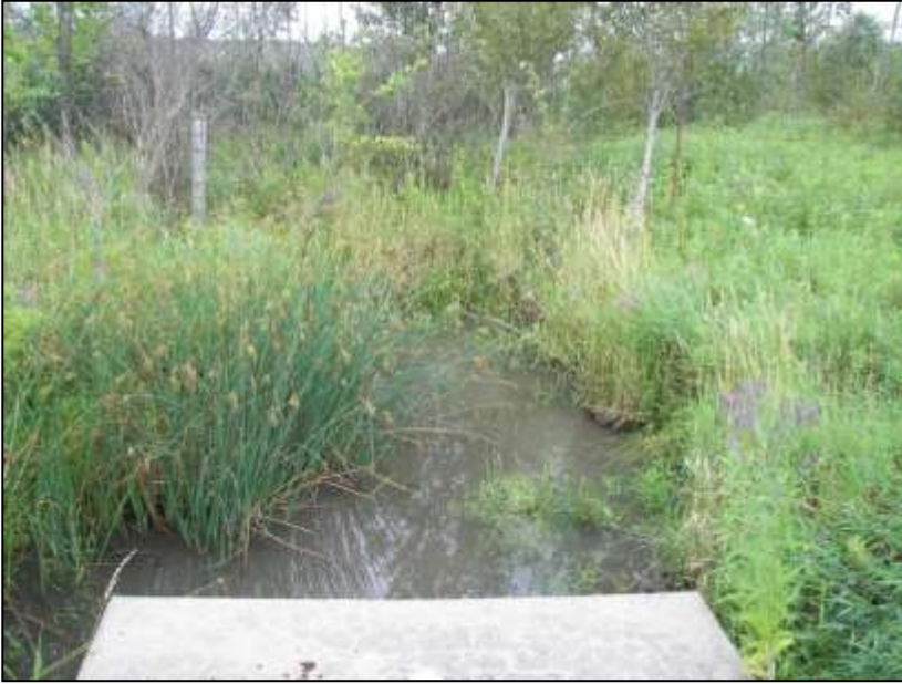
Runoff from Hwy 115 at Cell A.
