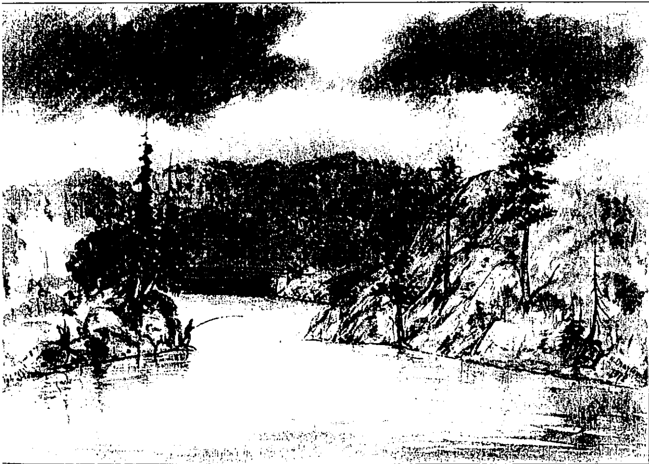
40. "Burleigh Bridge and Chute," Drayton 1878, Archives of Ontario
