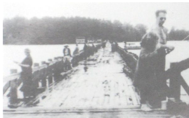
Figure 11: Chemong Floating Bridge in the 1930s. (Source: The Holy Land: A History of Ennismore Township )
