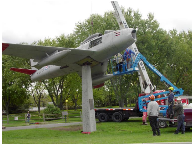
Figure 6: Removal of Jet. (Source: Bob Ough)
