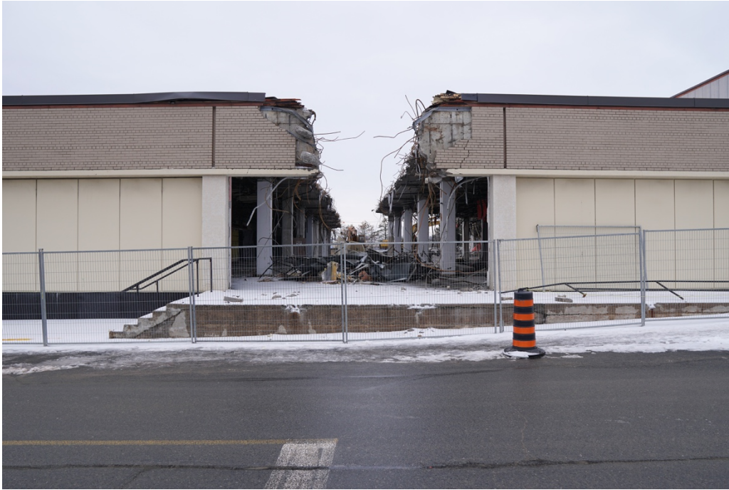
Photograph of the demolition of Sears department store in Peterborough Ontario.
