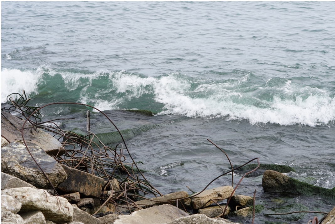
2017-10-09 | Rebar in the water at one of the shorelines.
