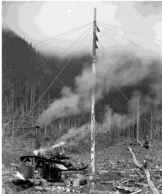
Fig 32. A spar tree in a Green Point Logging Co. Ltd. logging operation (August 1932). 629
