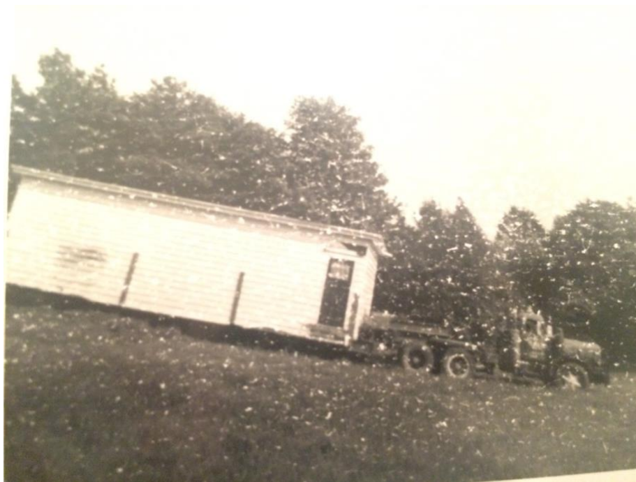
Figure 20 - The school portable, purchased by Ferguson, being trucked the last few hundred yards up the hill to its final position. By permission of the Ferguson family.
