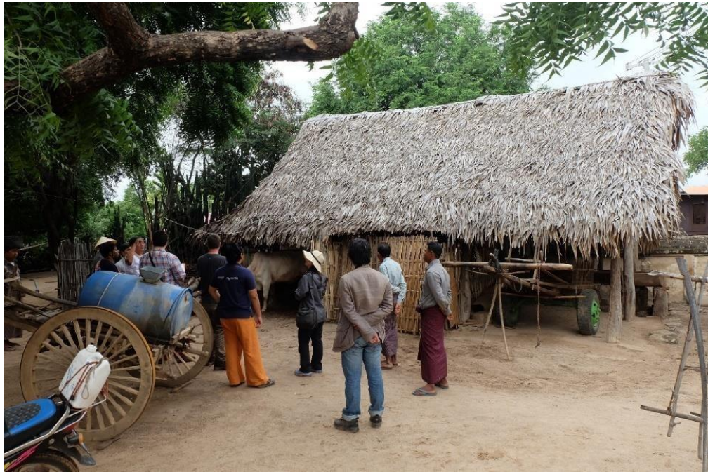
Figure 4.3. Southern side of cow shed (Courtesy of Talis Talving-Loza and IRAW@Bagan Project).
